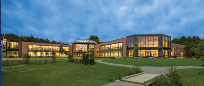
Hamilton Storage Headquarters
